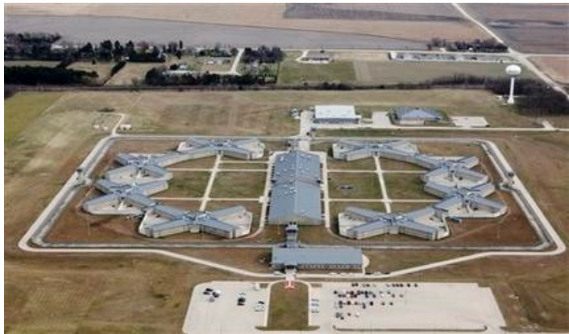
Luftbild des Thomson Correctional Centers in Illinois (AP Foto: Charles Rex Arbogast)
